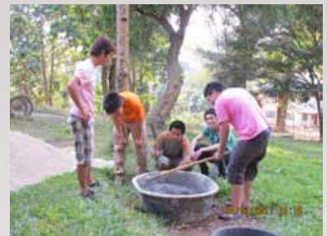
Chaplain Apirak is supervising students mixing cement.
