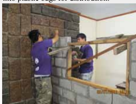
Piyanut and Vorachat are laying blocks for a radio studio.
