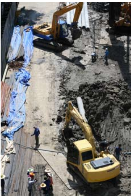
Two backhoes excavating the construction site
