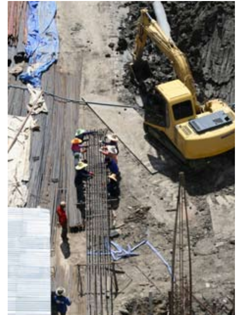
A backhoe is excavating the construction site
